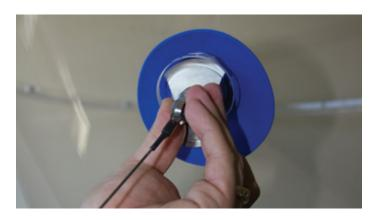
5. Install Fast-Fit™ alignment plate onto the retaining cable (or pipe) and into the bin with the shoulder positioned outward. Center the alignment plate in the mounting hole, aligning it in the vertical position with the arrow pointing upwards.
