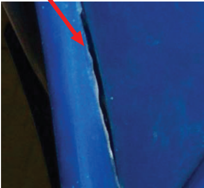
CRACKS Inferior geometric design
